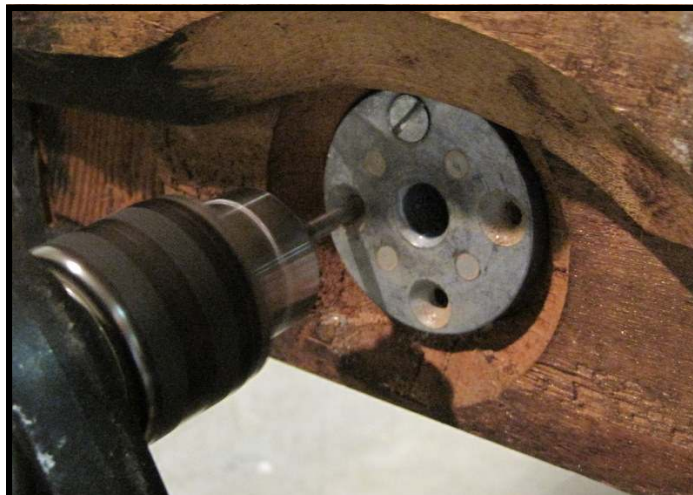
New socket being installed.
